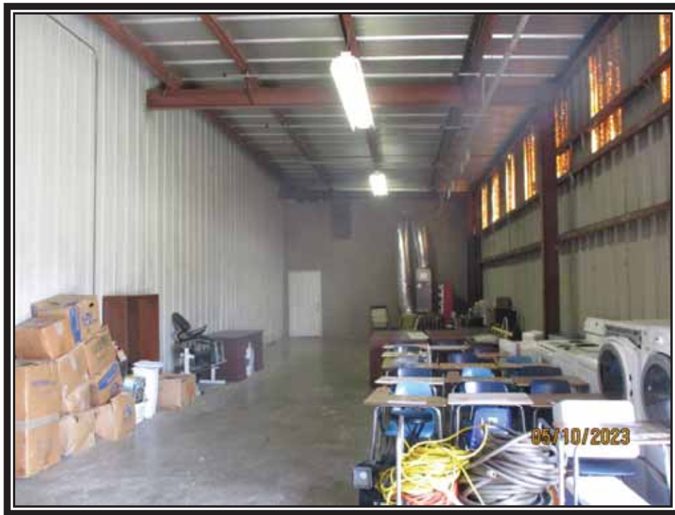
Interior View of Non-Conditioned Warehouse Space
