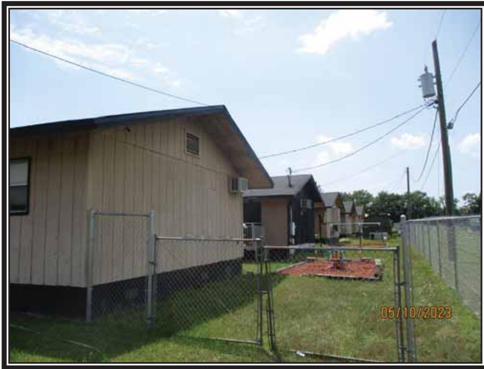
Exterior View of Childcare / School Building
