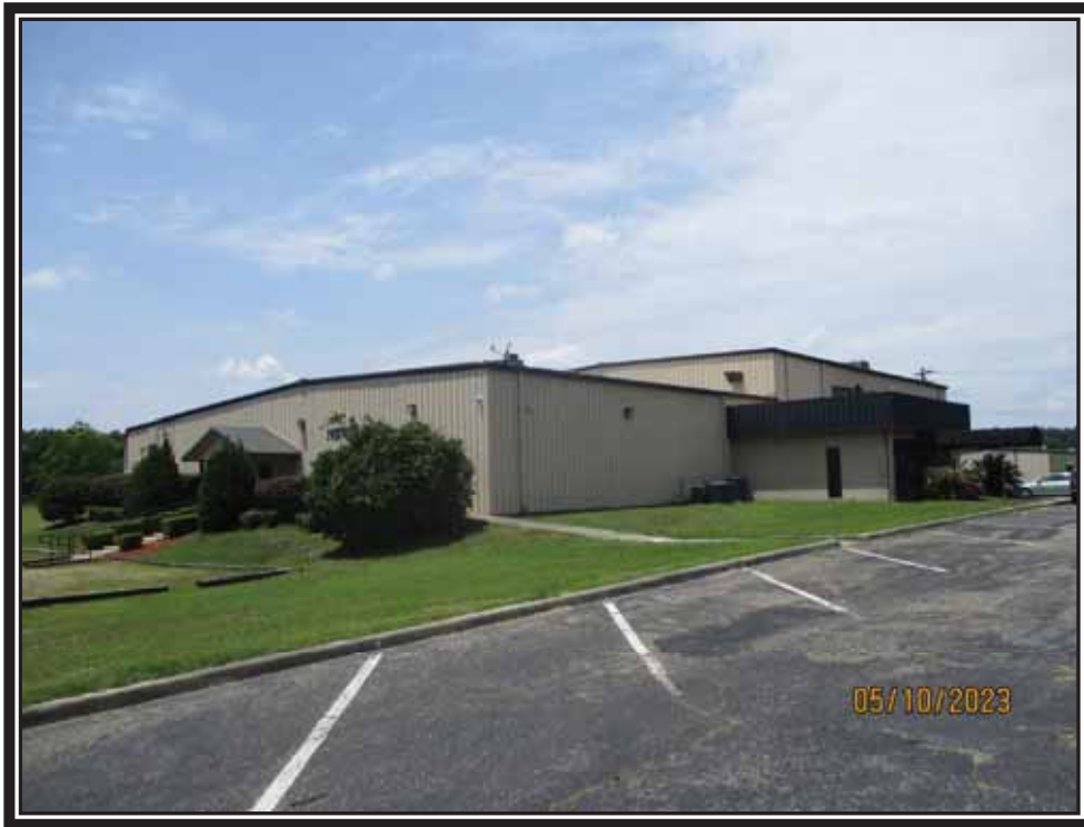
Exterior View of East & South Elevations of Sanctuary Building
