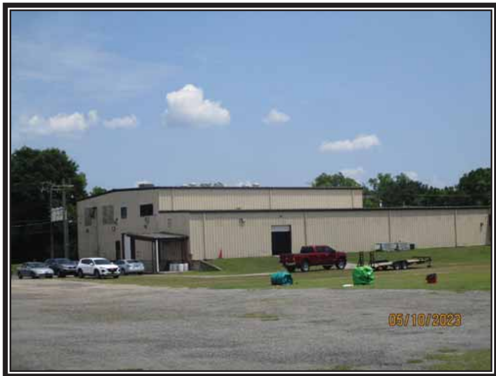
Exterior View of North & West Elevations of Sanctuary Building
