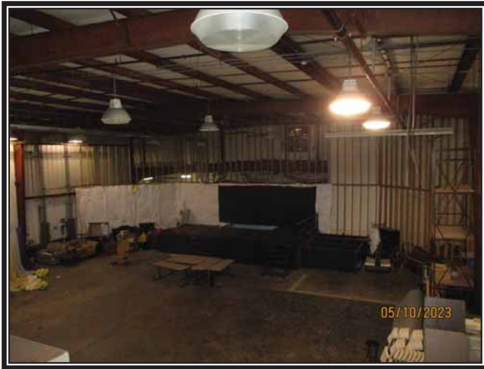
Interior View of Conditioned Warehouse Multi-Purpose Space
