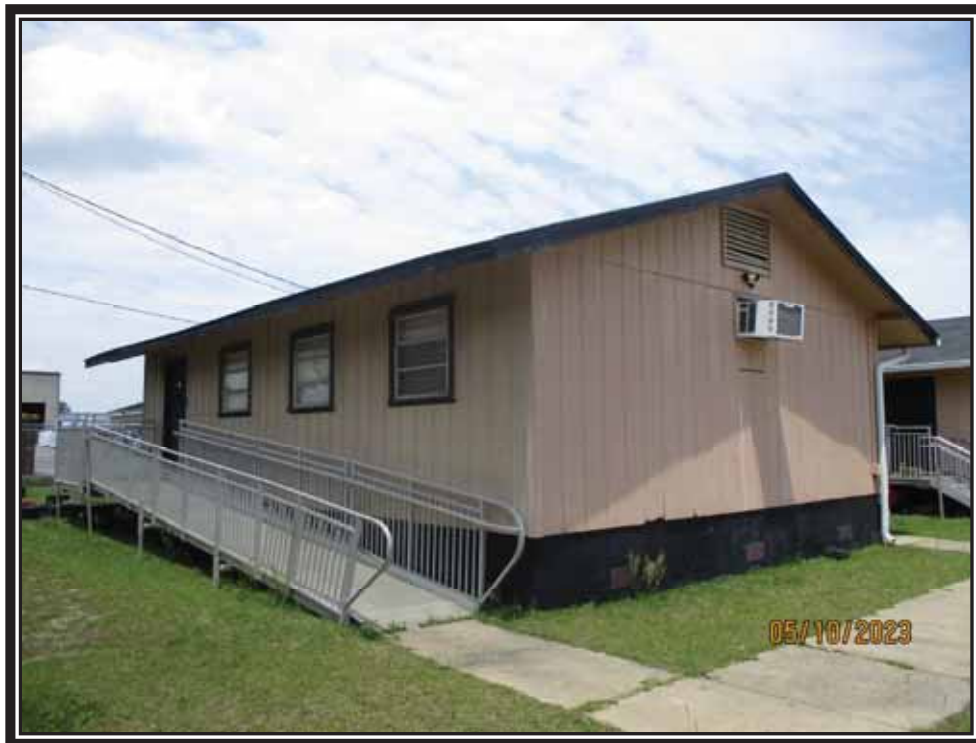
Exterior View of Childcare / School Building
