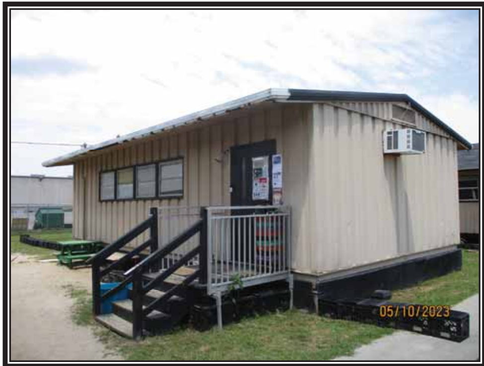
Exterior View of Childcare / School Building
