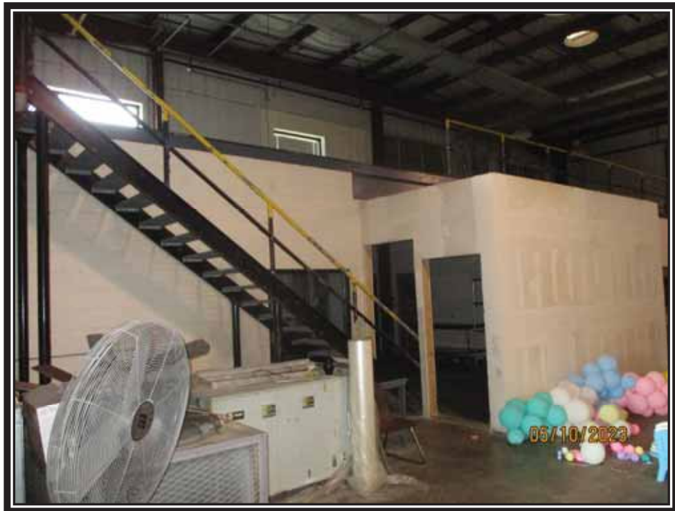
Interior View of Conditioned Warehouse Multi-Purpose Space
